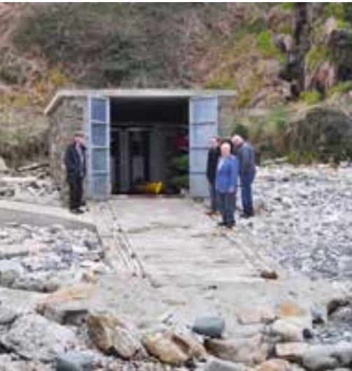
▲ Renovated boat shed for kayaks at Fort Dunree.
