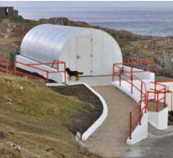
▲ The new interpretation centre at Fanad lighthouse.
